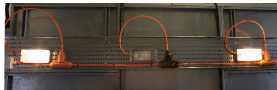
Connecta maintains the integrity of a circuit even if a local device suffers fire damage.
